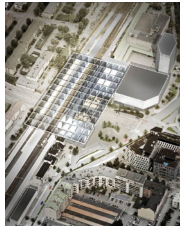
The two Örebro Stations: (far left) the artery connecting the two stations and proposals for Örebro Central station (left and below)
